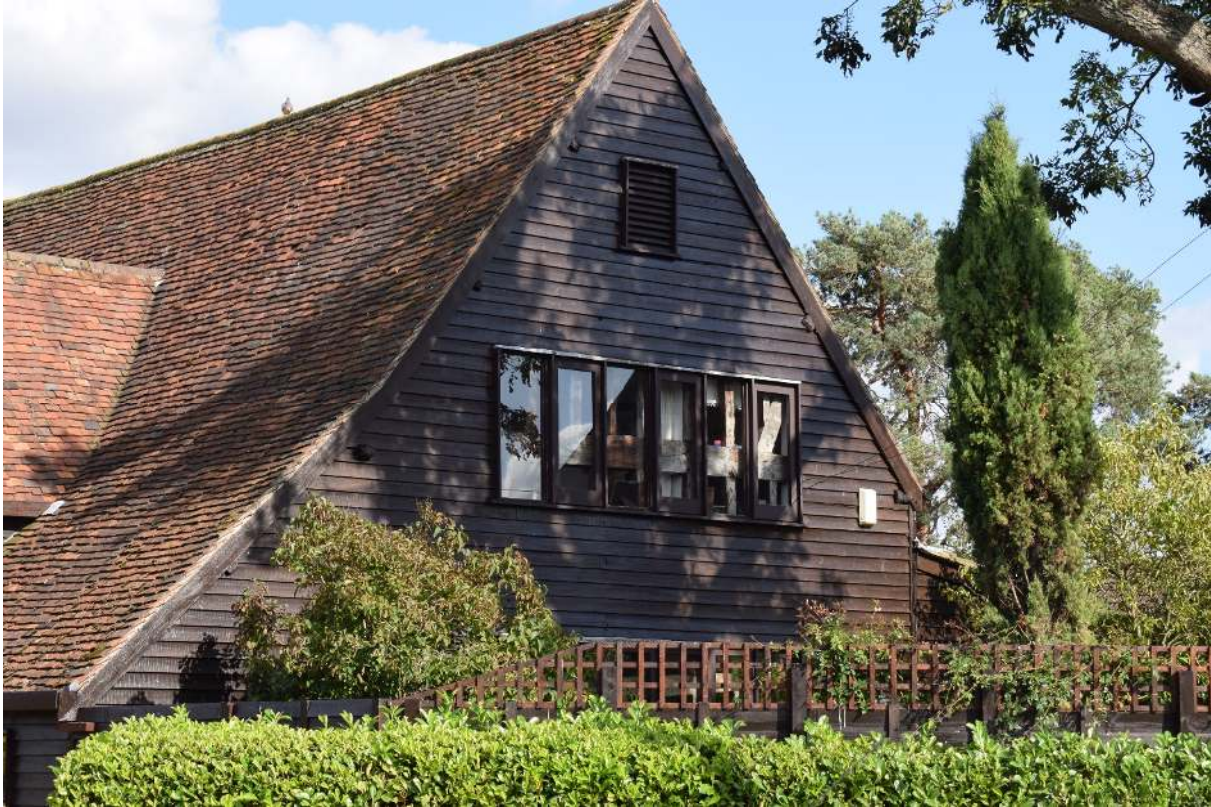
Figure 2.3: Timber framing visible inside Tythe Barn, off St Albans Road, grade II, NHLE 1347252.
