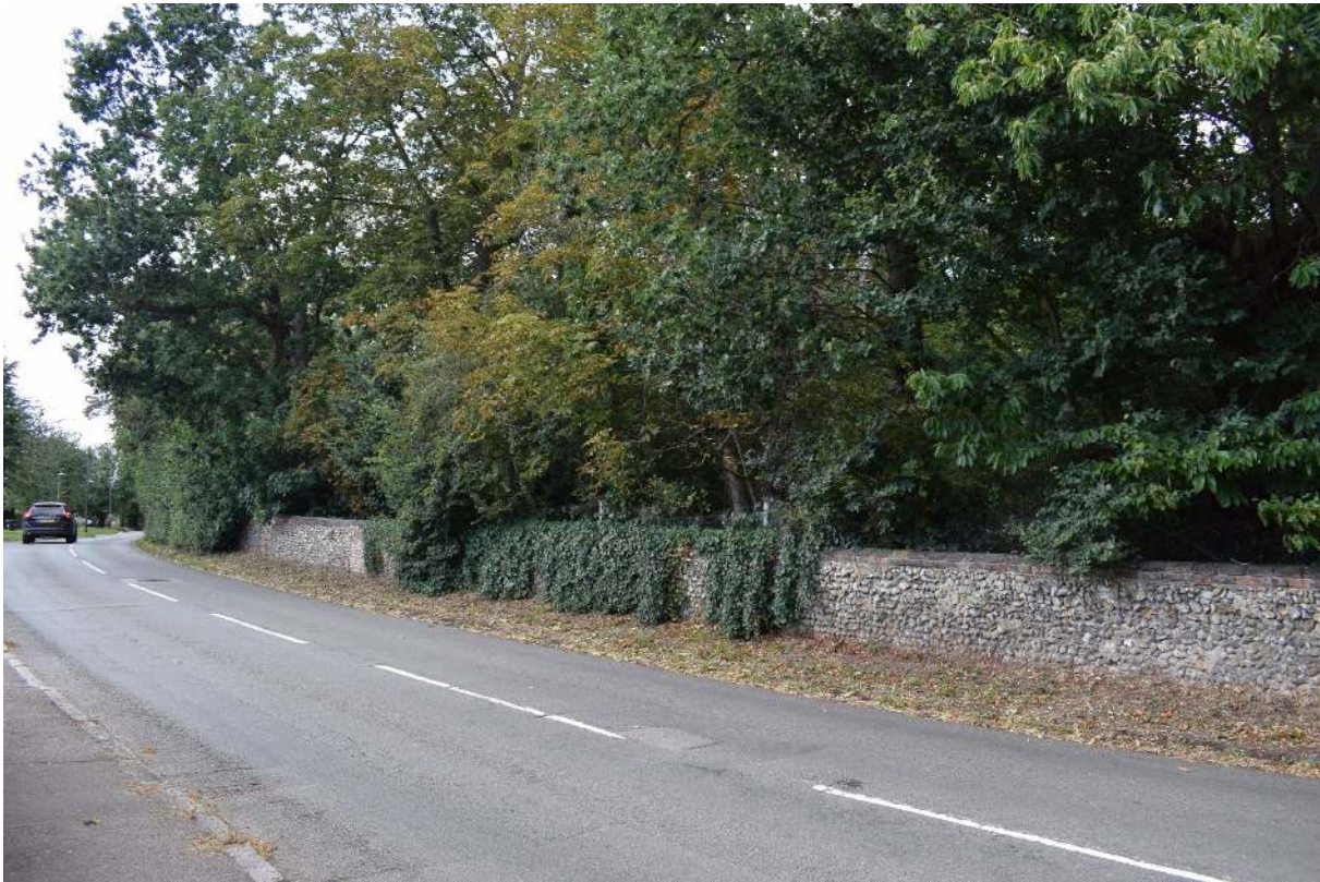
Figure 2.1: Walls of Codicote Lodge along Heath Lane showing the boundary of the Codicote Lodge estate
