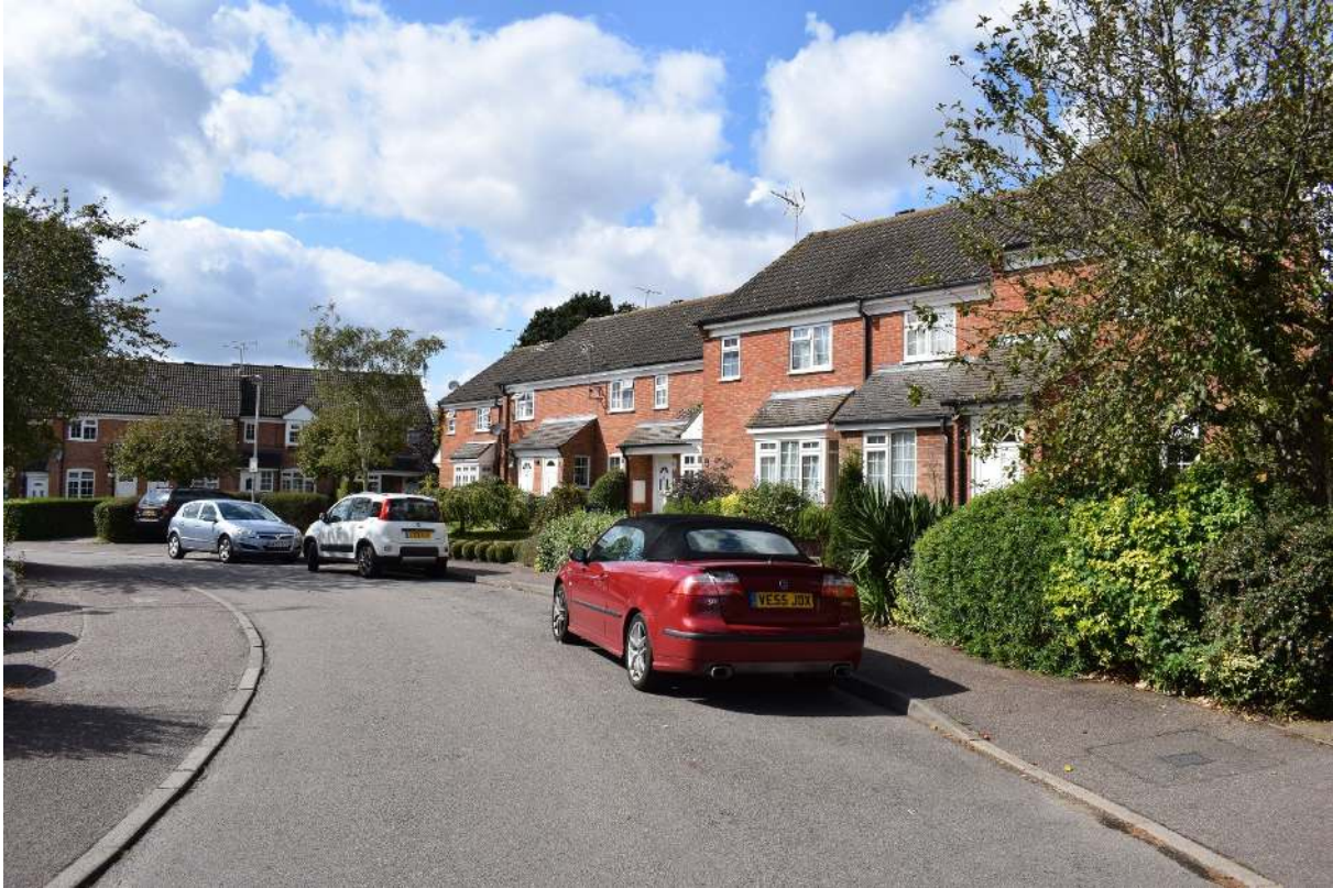
Figure 2.2: Old School Lane development, c. 1980s, a modern development with character at odd with the rest of the Conservation Area
